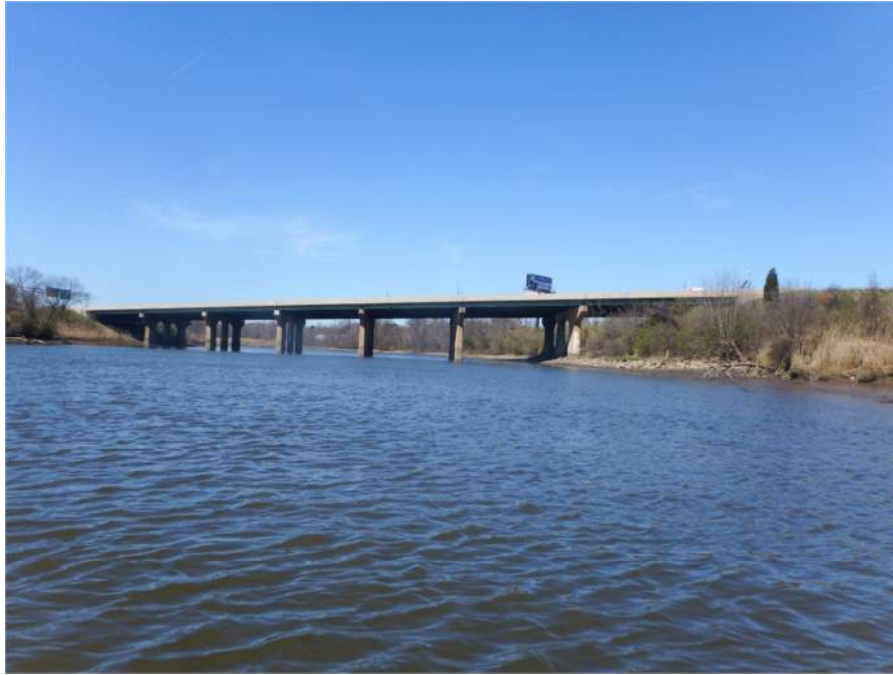
Photograph 1. Overall View of the East Elevation, Looking West.
