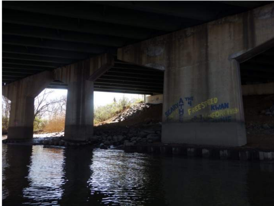
Photograph 3. Typical Configuration of Pier (Pier 1 shown), Looking Southeast.
