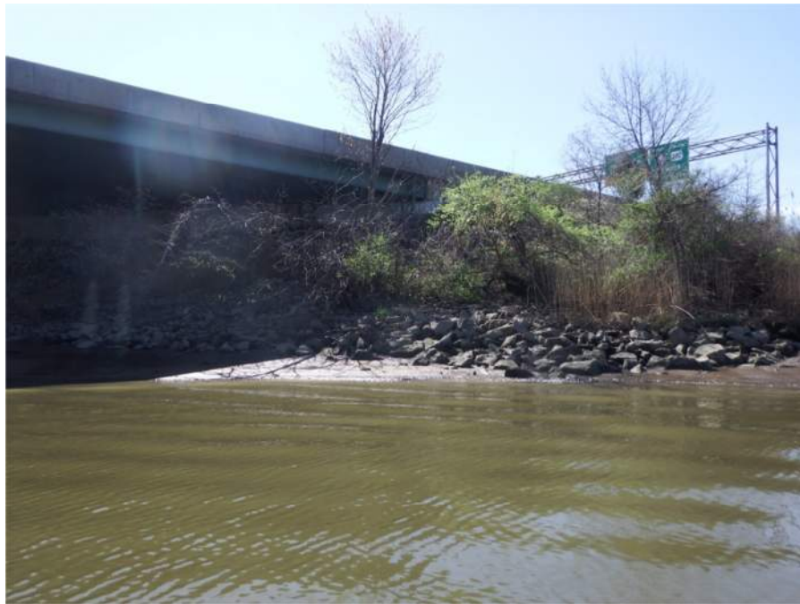
Photograph 7. Typical View of Embankment (Southwest Shown)
