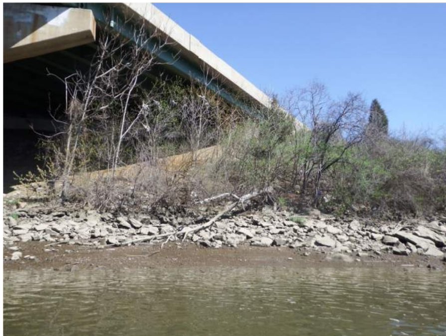
Photograph 8. Typical View of Embankment (Northeast Shown)
