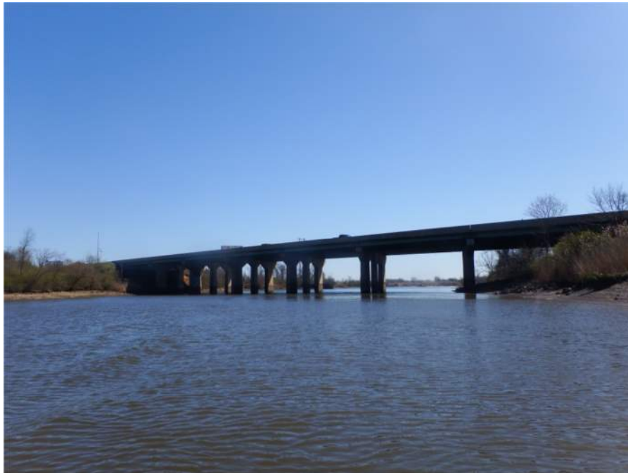
Photograph 2. Overall View of the West Elevation, Looking East.
