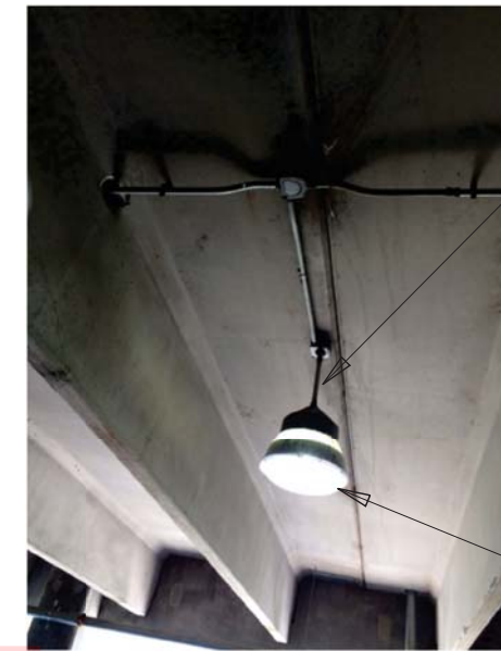
EXISTING LIGHT FIXTURE MOUNTING
