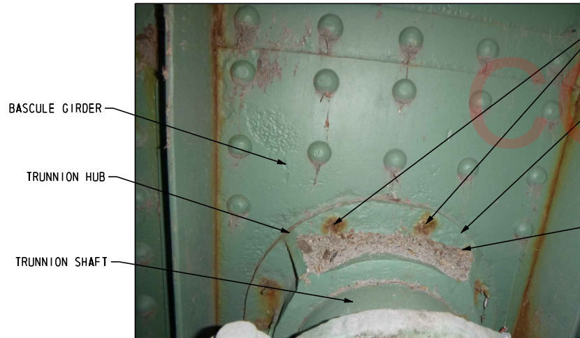
WEST TRUNNION ASSEMBLY - INBOARD SIDE
