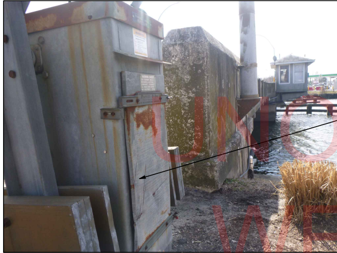
DAMAGED REAR DOOR AT THE NORTH WARNING GATE
