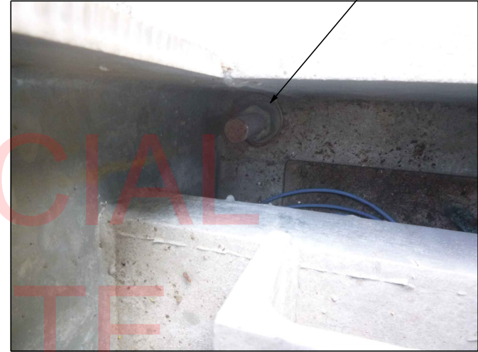
LOOSE ANCHOR AT THE BASE OF THE SOUTH WARNING GATE
