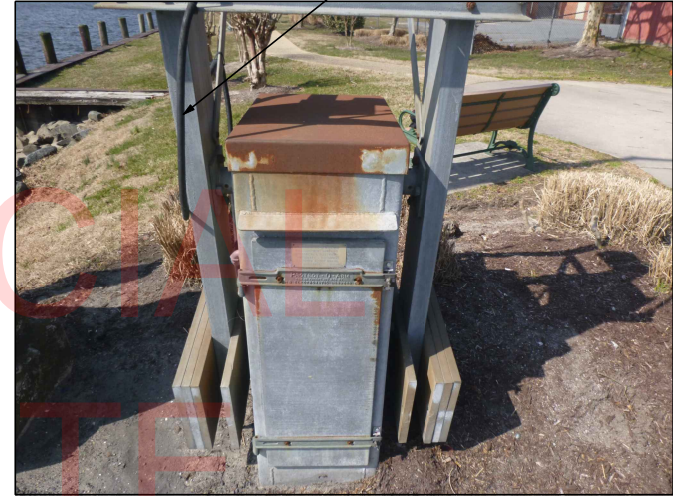
DAMAGED SOW CABLE FOR THE NORTH WARNING GATE FLASHER
