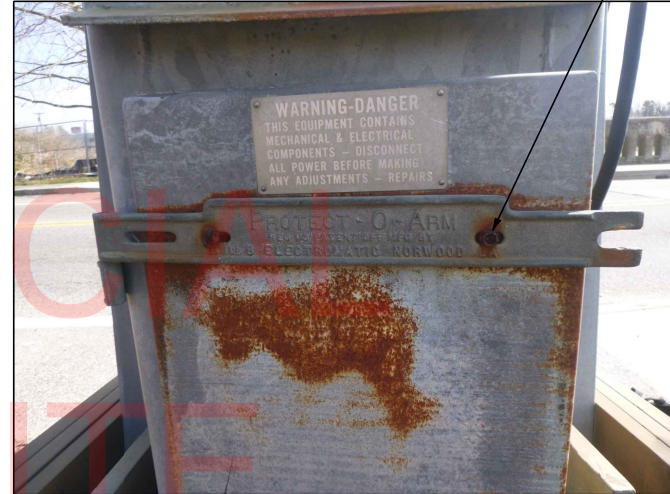
TYPICAL CORRODED HARDWARE ON THE NORTH WARNING GATE DOOR STRAP
