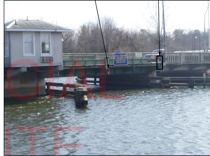
TYPICAL SPAN MOUNTED NAVIGATION LIGHT LOCATED AT THE CENTER OF THE SPAN
