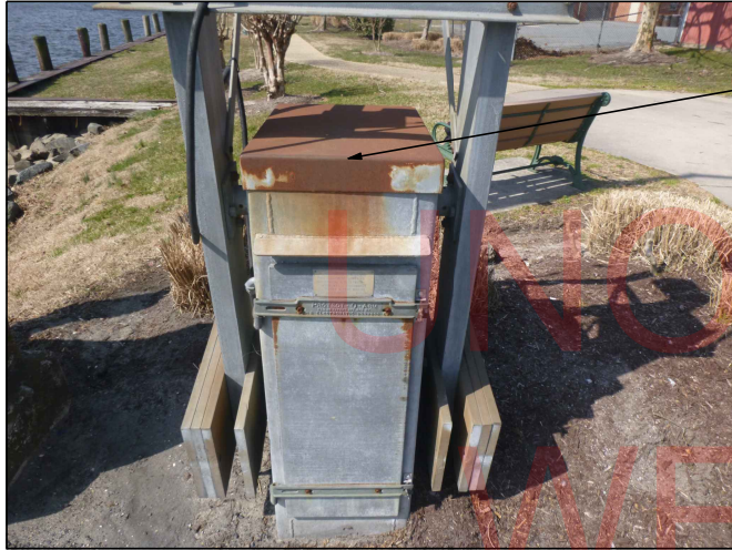
NORTH WARNING GATE HOUSING WITH CORROSION
