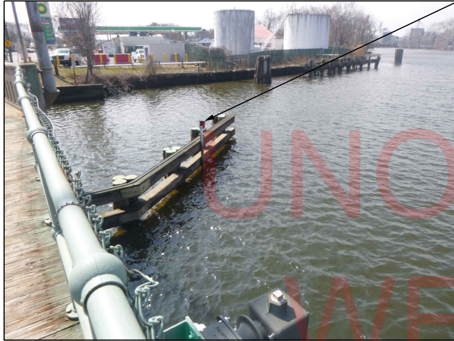
TYPICAL FENDER PIER LIGHTS NOT ALIGNED WITH THE CHANNEL
