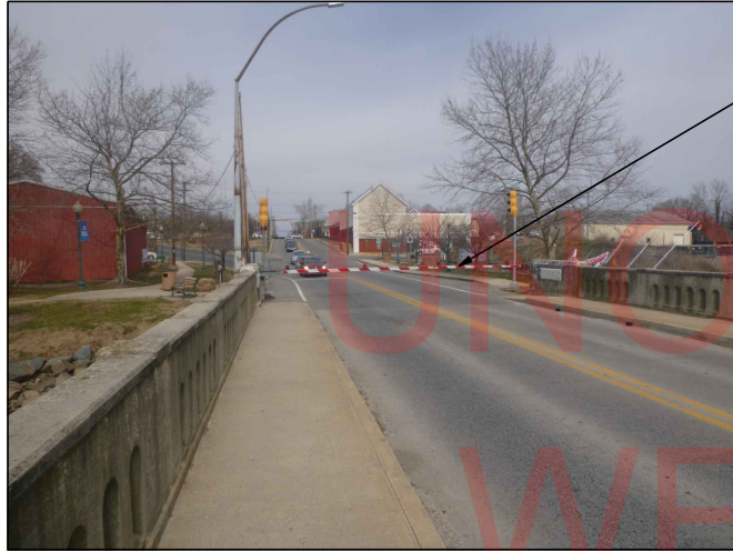
NORTH WARNING GATE ARM WARNING LIGHTS NOT IN COMPLIANCE WITH THE MUTCD
