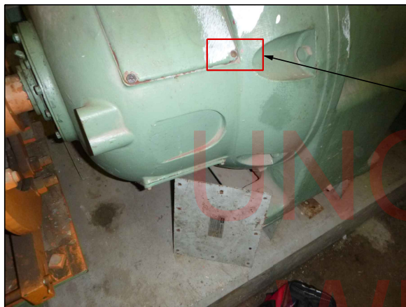
TYPICAL SPAN MOTOR WITH MISSING HARDWARE ON ACCESS COVER
