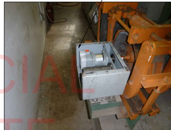
TYPICAL TACHOMETER AND OVERSPEED ENCLOSURE WITH UNSECURED COVER (2 TOTAL)
