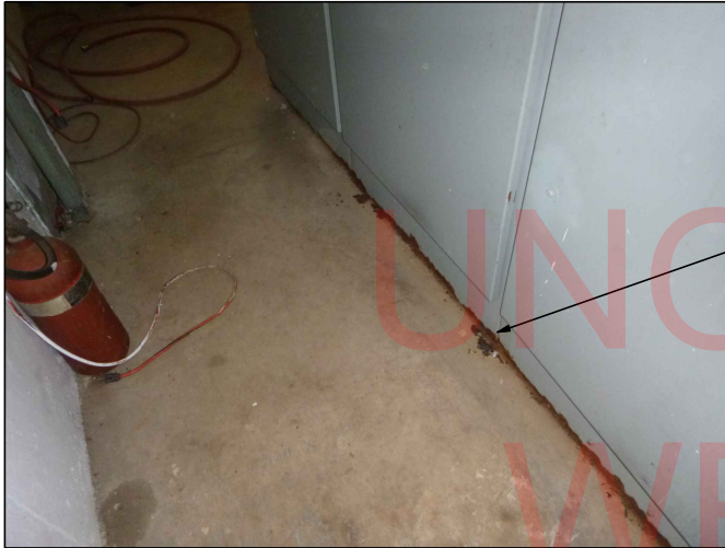
TYPICAL CONTROL ENCLOSURE WITH CORROSION AT THE BASE
