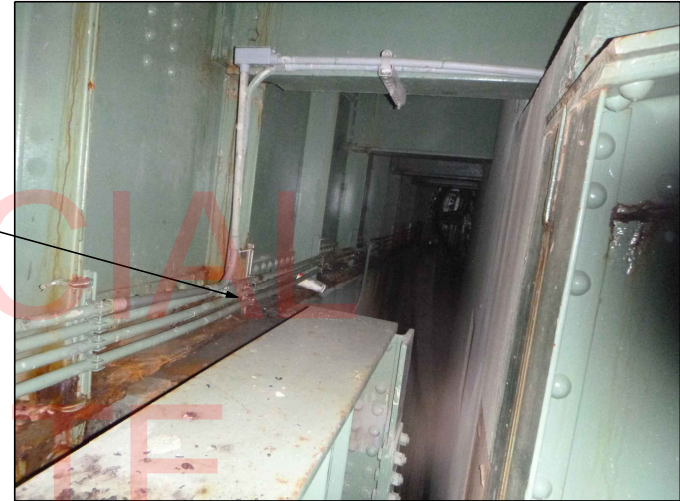
TYPICAL CONDUIT IN BASCULE PIER WITH PEELING PAINT AND CORROSION
