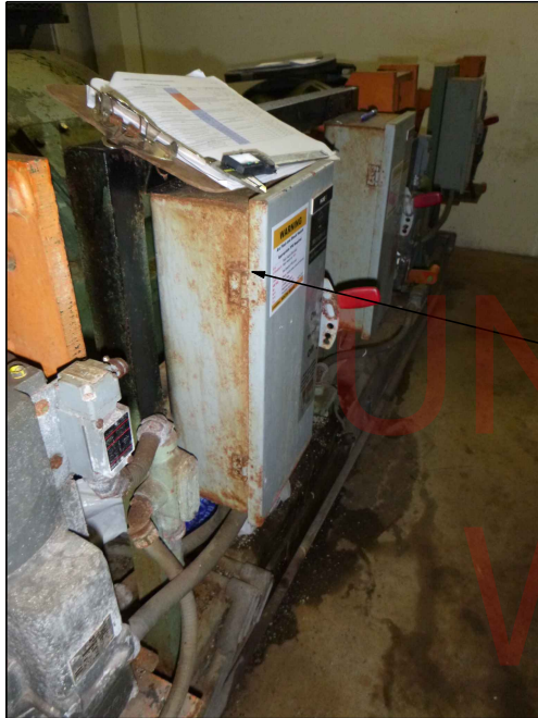
TYPICAL MOTOR DISCONNECT SWITCHES, CONDUIT AND FITTINGS WITH CORROSION
