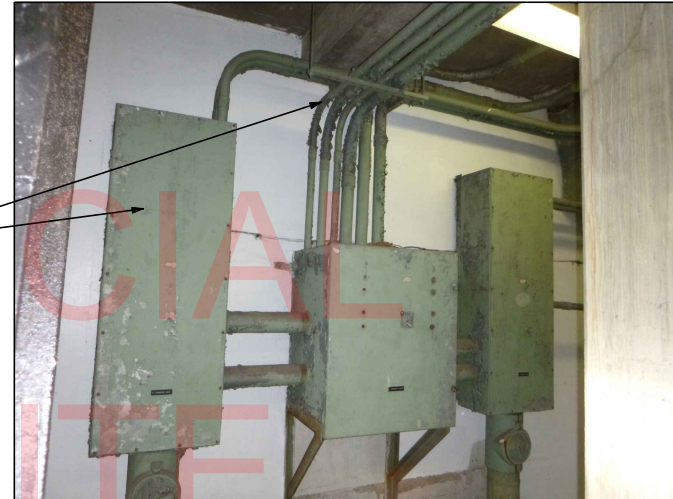
TYPICAL TERMINATION ENCLOSURES, CONDUIT AND PULL BOXES EXHIBITING PEELING PAINT
