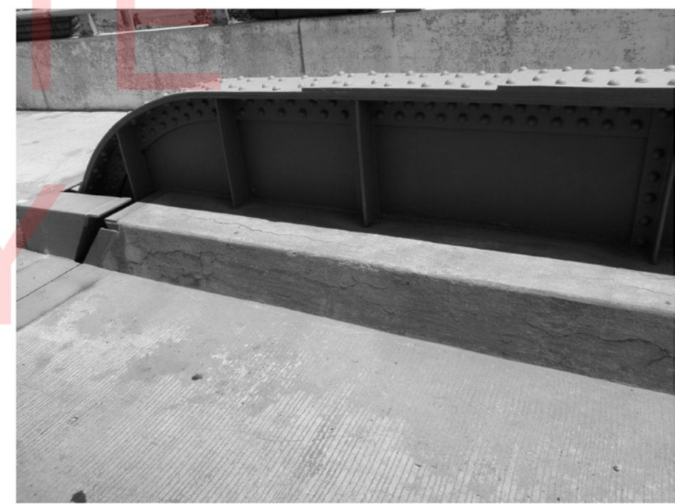
PHOTO 2 TYPICAL BASCULE GIRDER AT ROADWAY LEVEL NEAR HEEL JOINT
