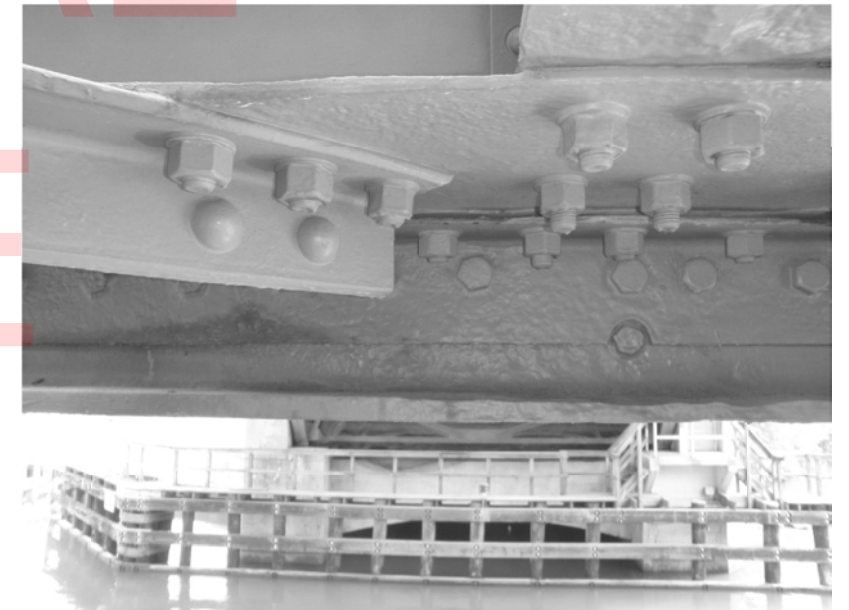
PHOTO 2 NOT TO SCALE NOTE: CLEAN & PAINT ALL EXPOSED SURFACES OF BRACING CONN. AT MIDSPAN OF FB USING THREE COAT SYSTEM; REFER TO TYP DETAIL ON THIS SHEET.
